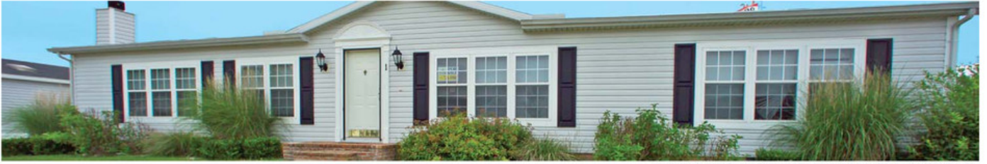
Community Photo from: East Fork Crossing - Batavia, OH
